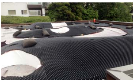
The planting areas were equipped with Floradrain® FD 40-E-elements while Floradrain® FD 60 was used as a base for the tree planters.
