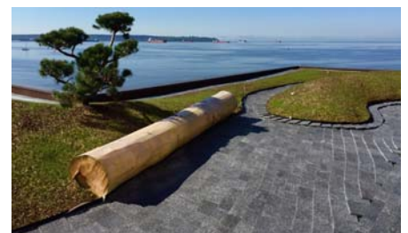
The walking areas were edged with angle profiles; Tree trunks serve as design elements.
