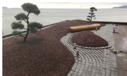
Square-shaped slabs form the walkways on the roof surface.
