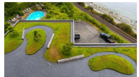
Features like topiaries and tree trunks provide accents on the roof. The illumination behind the angle profiles is visible only in the dark.
